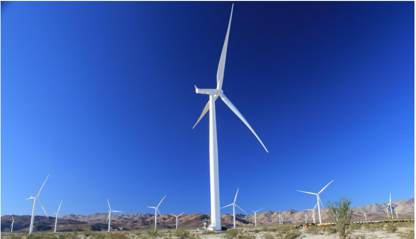
Figure 5 show the Ocotillo Express Wind Energy Facility in February 2013 while part of the farm was still under construction. Note the coils of copper wire to the right in the foreground. The controversies have not gone away, but some studies suggest that local views toward wind power are more positive over time.
