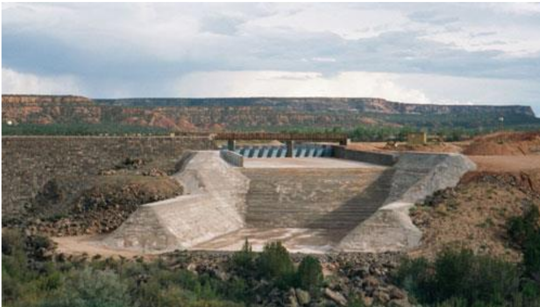
The Black Rock Dam in the Zuni Irrigation Project
